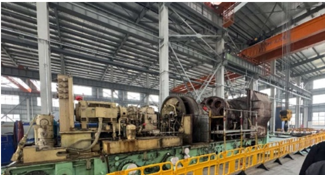
GE Frame 6B Unit — Pre-Overhaul Inspection
